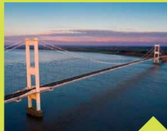
M48 Severn Bridge
